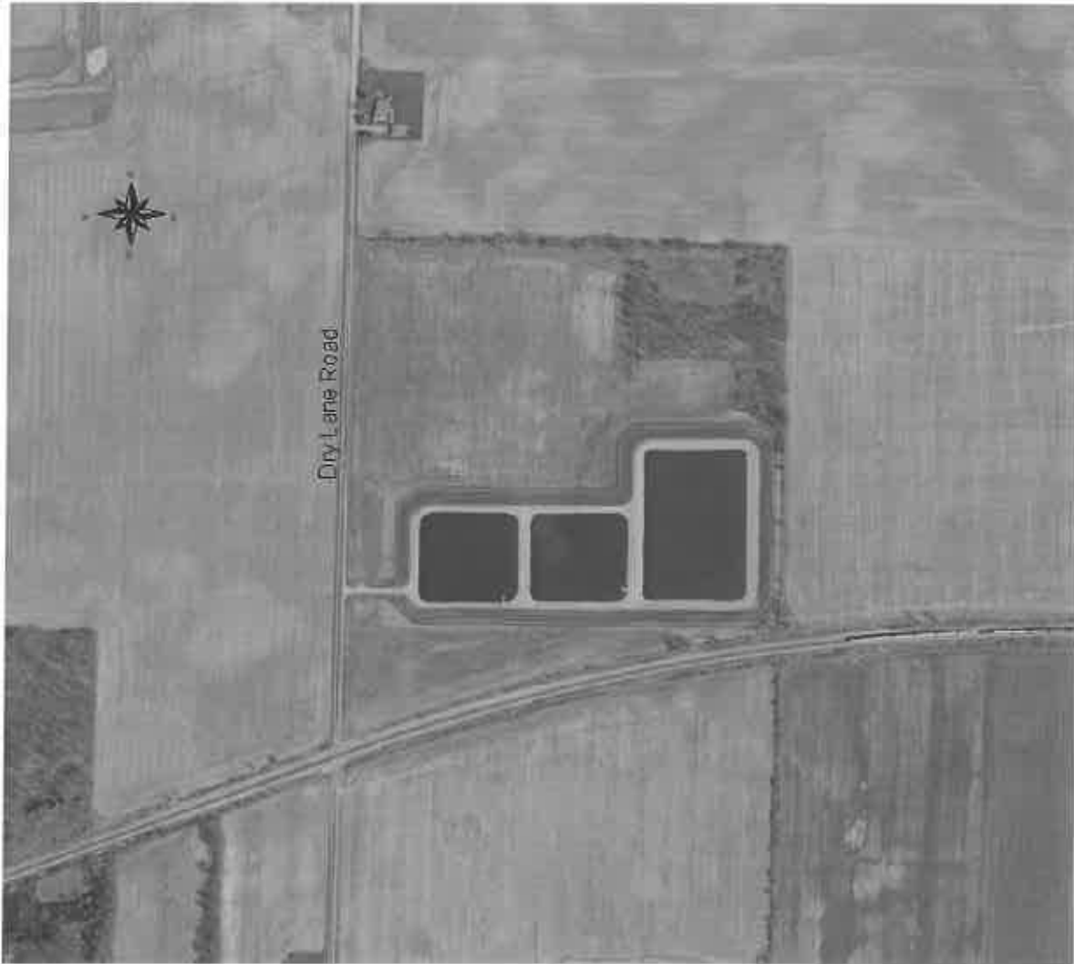
Figure 4 LaRue Wastewater Treatment Plant
